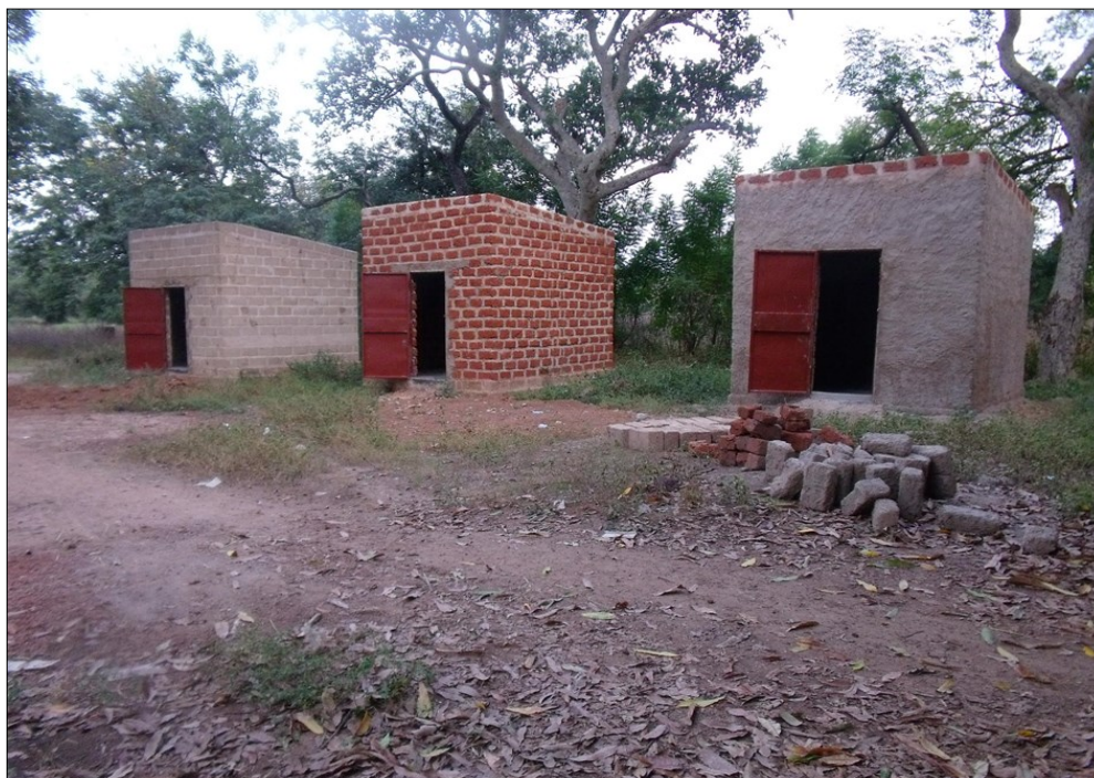
Figure 1. The concrete stone house, the red-stone house and the mud-house dimension 2.5 x 3 m in ground area.
